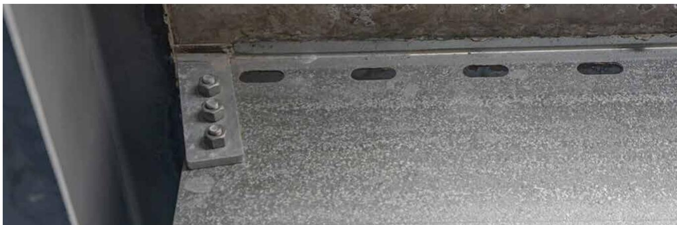
The durability of a galvanised coating is dependent on the thickness of the zinc coating, the general environment and the level of maintenance carried out over the life of the product. Consideration must be given to these factors when specifying SPEEDFLOOR® to determine the longevity of the structural solution. Further clarification of protective coatings and corrosivity zones should be sought from AS/NZS2312:2002 and HERA Report R4 -133:2005.
